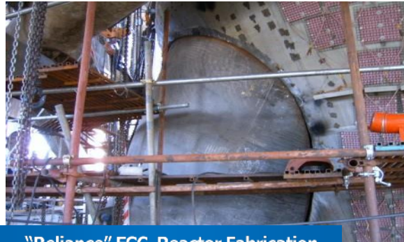
"Reliance" FCC Reactor Fabrication
